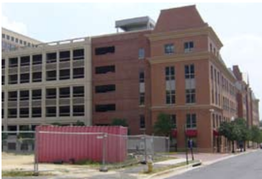
Separate structured parking from streets with occupied buildings, as in this example of housing built in front of parking in Alexandria, Virginia.
