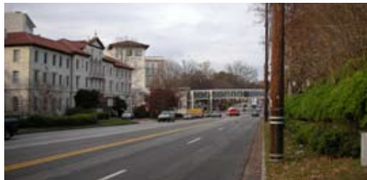
New development projects should repair discontinuities in the surrounding pedestrian network, such as at Houston Mill and Clifton roads (upper photo) and along Clifton Road near Gambrell Drive (lower photo).
