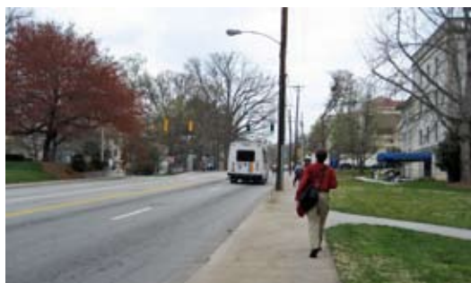
Existing utility poles less than 4' from the curb present a hazard to vehicles.
